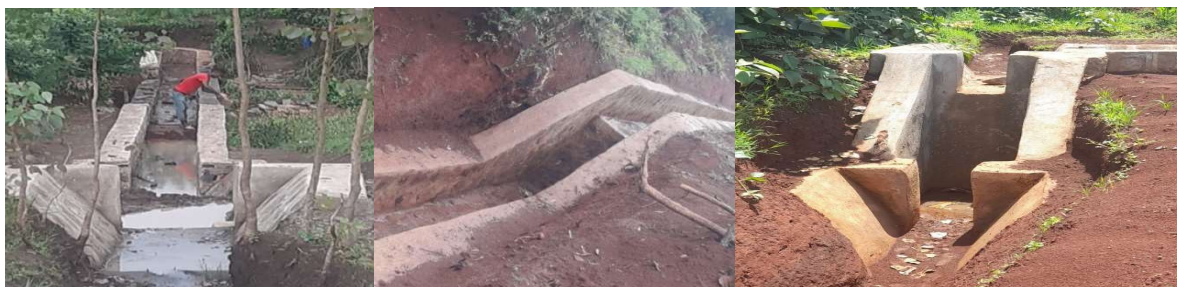
Figure 15: Drop Structures constructed
