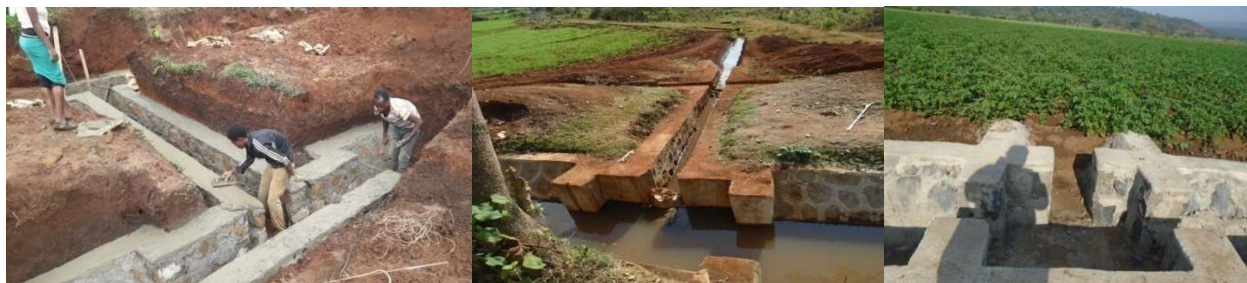
Figure 16: Division boxes constructed on main & Branch Canal
