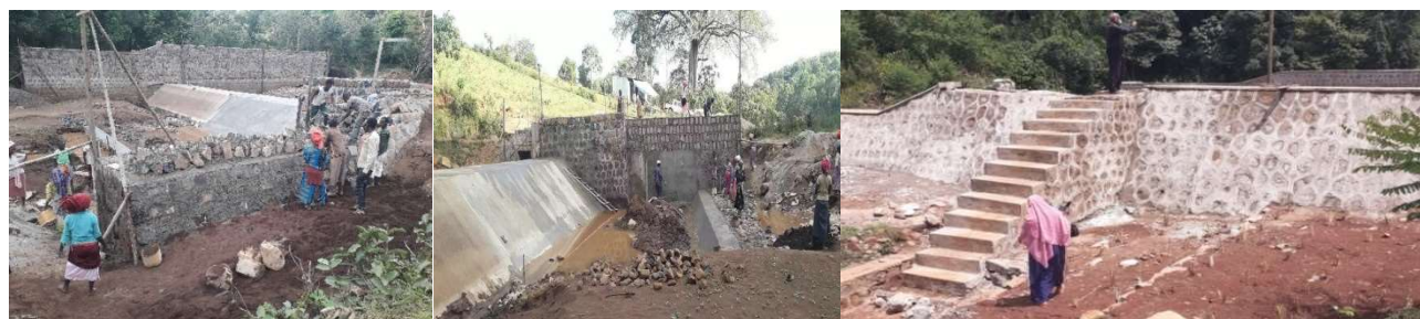
Fig 4: Retaining wall & walking stair completed
