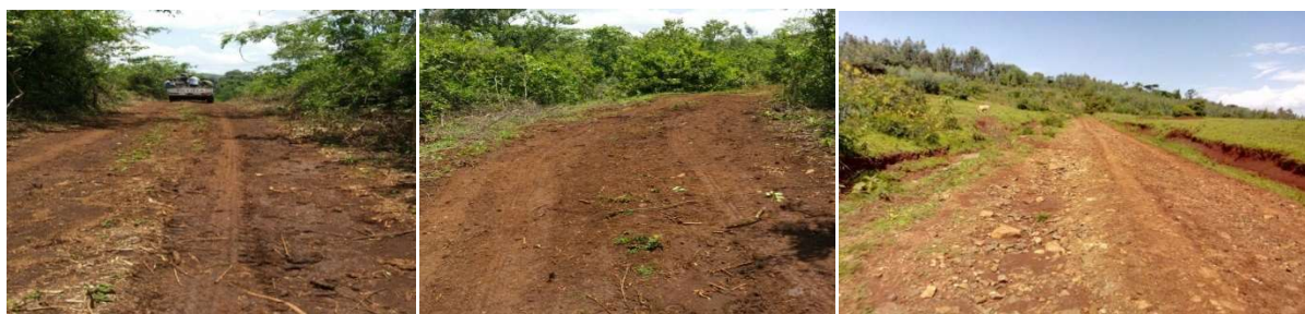
Fig 2: Access road maintained
