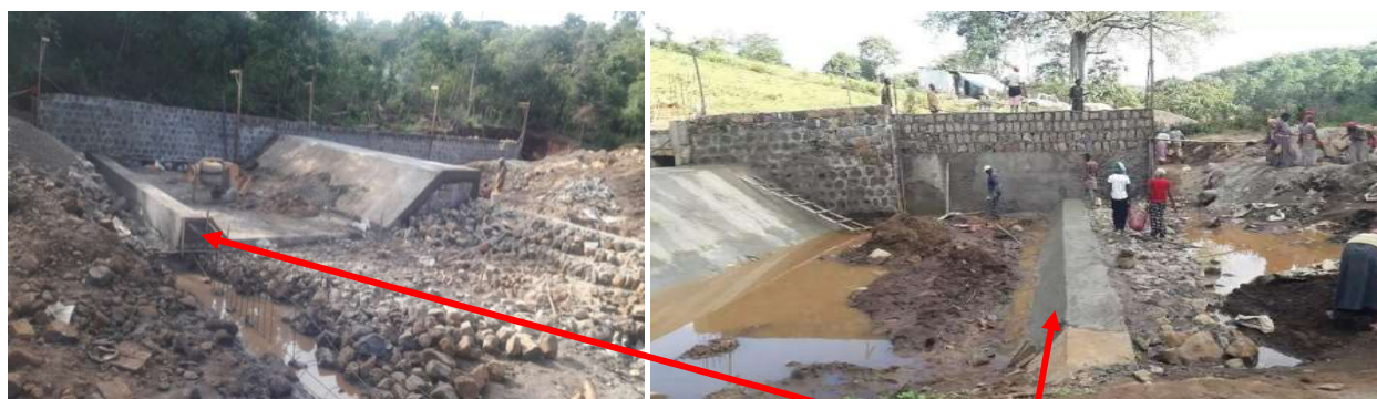
Fig 19: concrete end sill constructed
