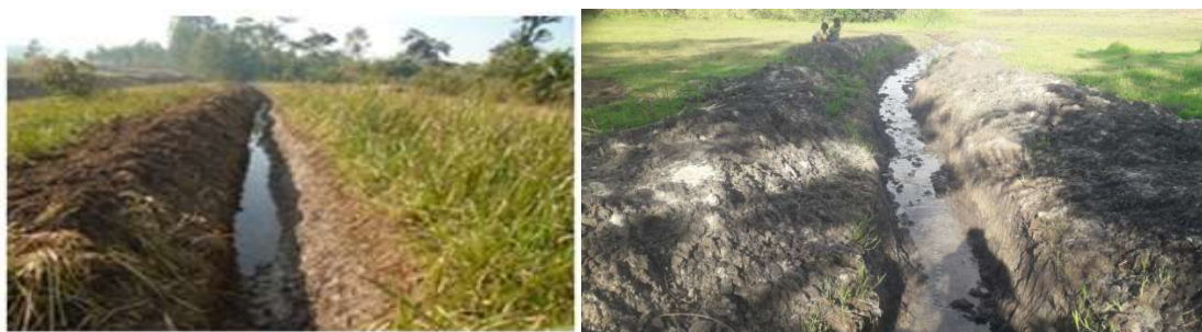
Fig 10: Drainage canals excavated
