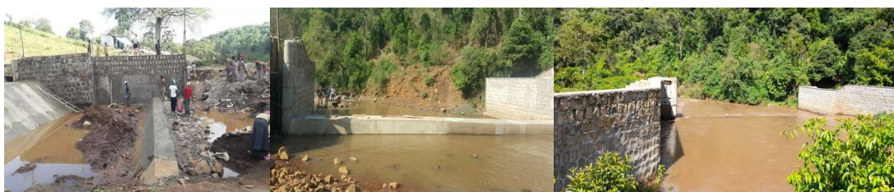
Figure 3: Weir body constructed & completed
