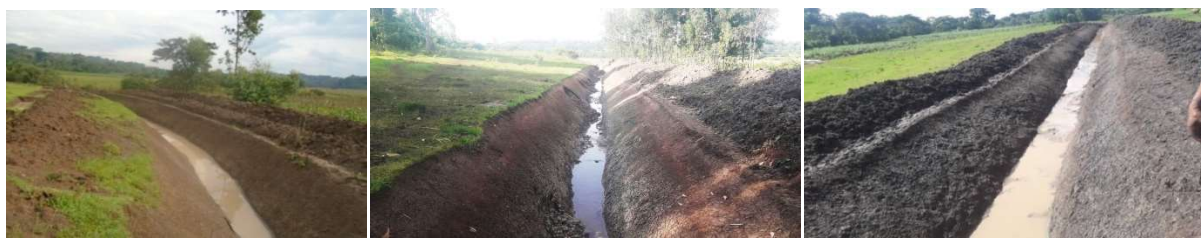
Figure 8: Branch Canals excavated
