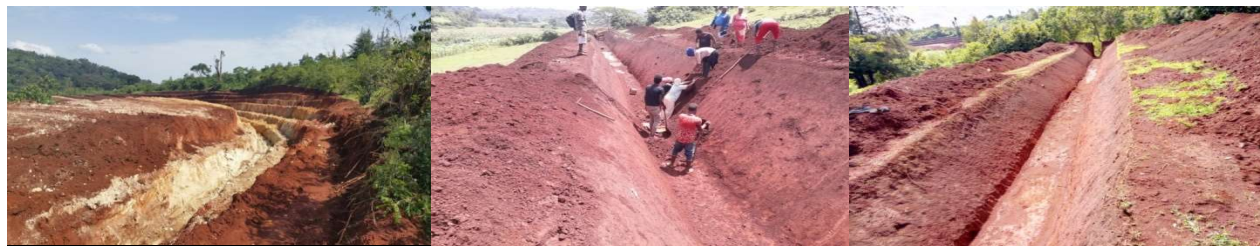
Fig 7: Main canal excavated by machine and human labour
