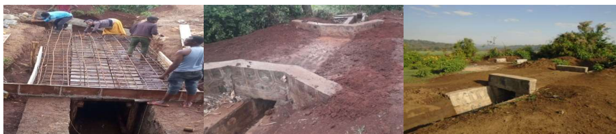
Figure 13: Completed Road culverts
