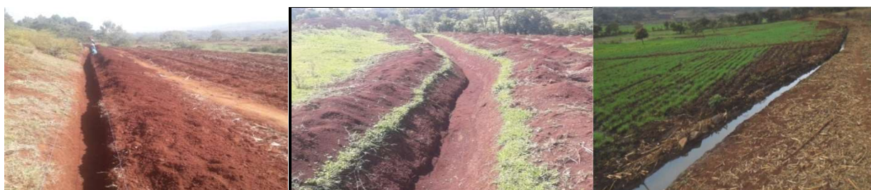
Figure 9: Completed Secondary Canal sections
