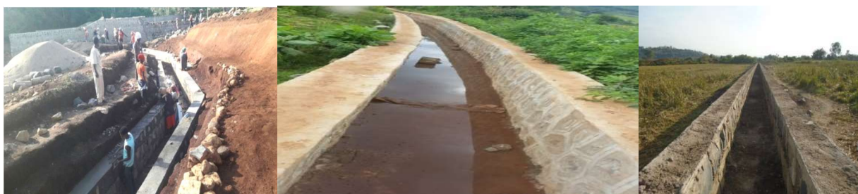
Figure 6: Lined canal constructed
