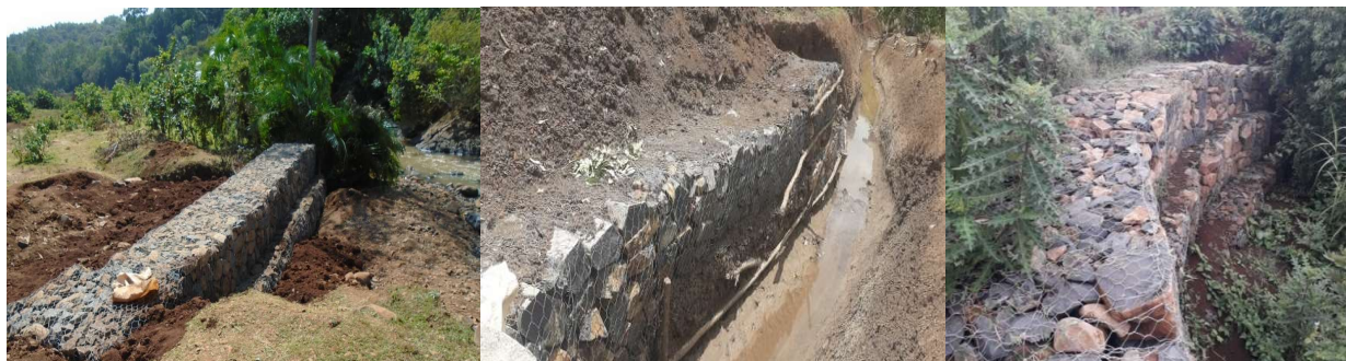
Figure 18: River Bank and canal embankment Protected by Gabion wire
