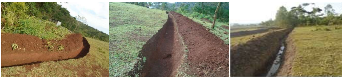
Fig 28: Cut off drains excavated above the canal areas
