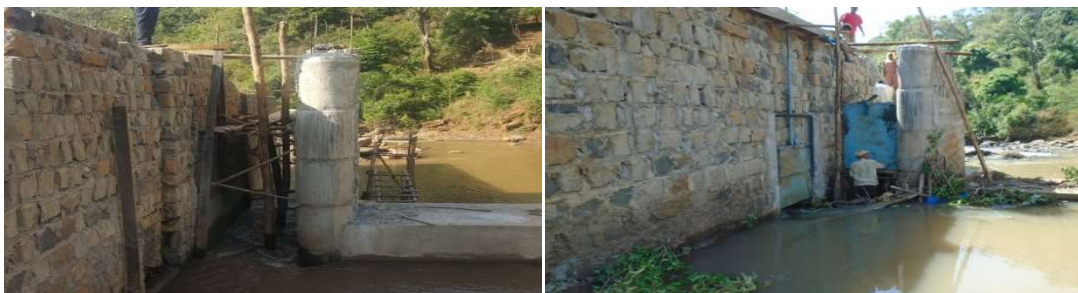
Figure 5: Divide wall constructed b/n retaining wall & weir body and sluice gate fixed
