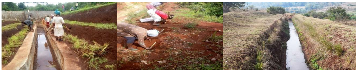
Fig 31: Vetiver planted at the canal and soil bund embankment
