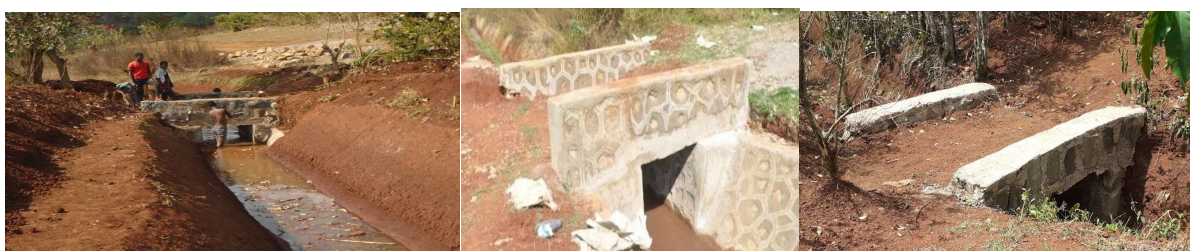
Figure 11: Completed Foot bridges
