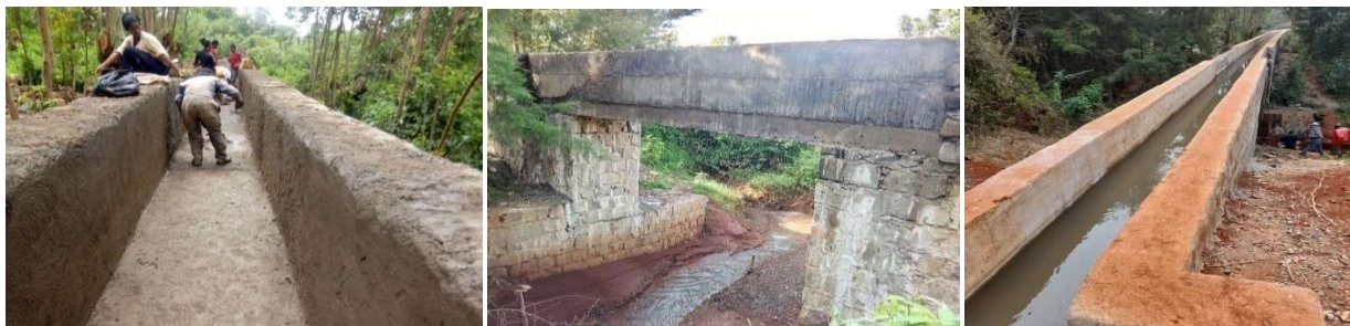
Figure 14: Drainage culvert constructed
